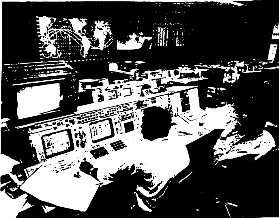
Figure 7.- Console of the Integrated Communications Officer in the Mission Contr Center.
